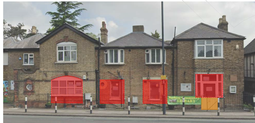
Lower existing window sill heights / insert windows to improve visual link to pedestrian route
